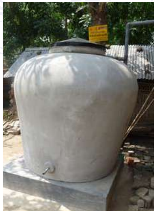
One of the RWH units completed in 2010. The rain water is collected from roof gutters and flowed into the unit via water pipes (top right). The community withdraws water from the tap (bottom left)
